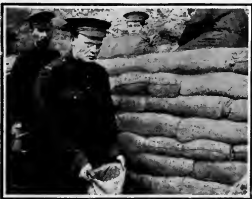
BUILDING A TRAVERSE IN A FRONT-LINE TRENCH.
